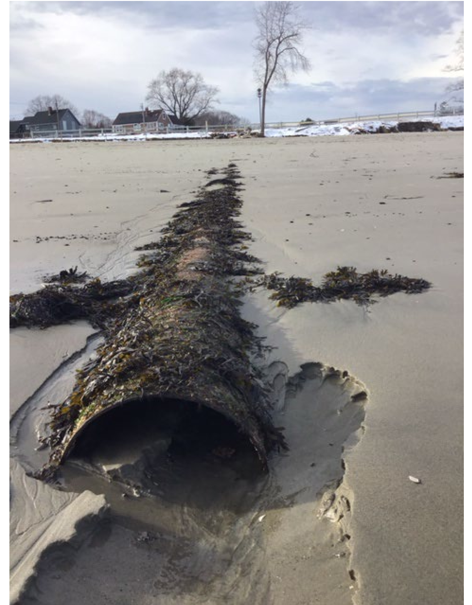
Stormwater Outfall On Willard Beach @ Ballfield
