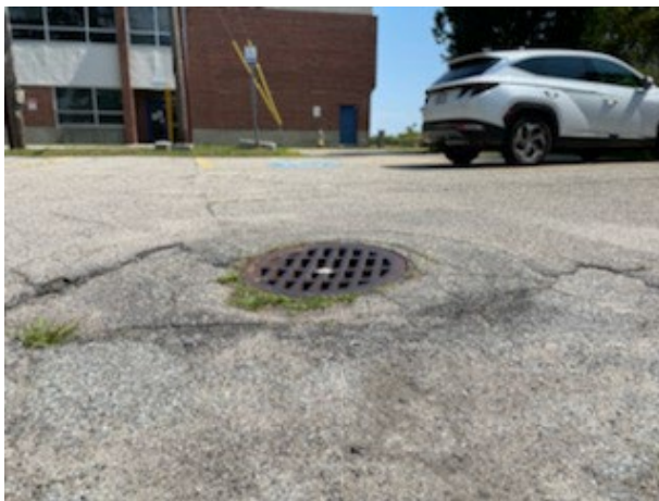
Photos above show CB_5013 before repairs and grate reset.
