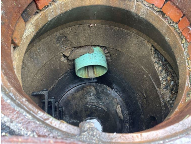
Above Left: BEFORE CB_5000 showing signs of deterioration. Above Right: AFTER CB_5000 concrete repaired
